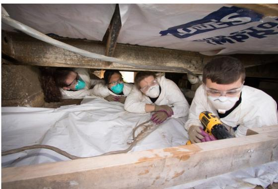
Volunteers work under a damaged mobile home to restore its foundation blocks and replace insulation
